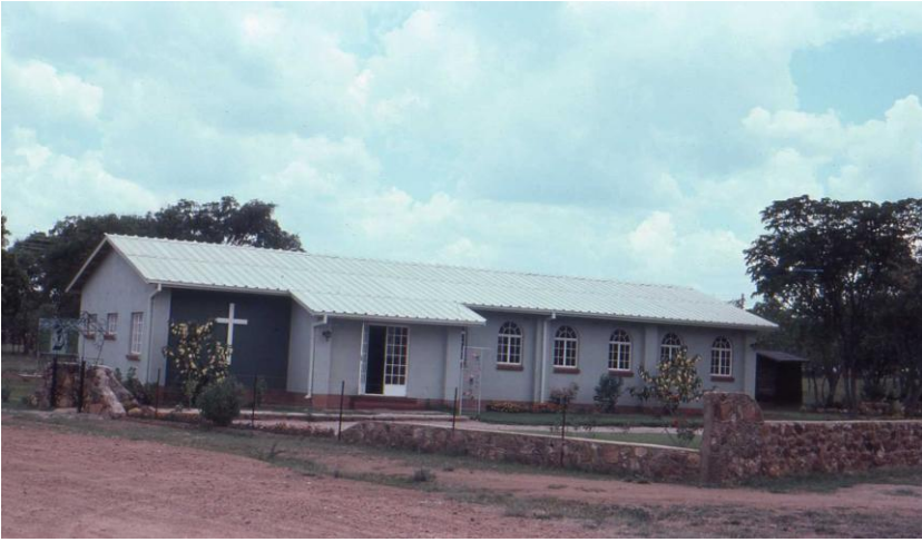
The church hall we built in Kwe Kwe.
