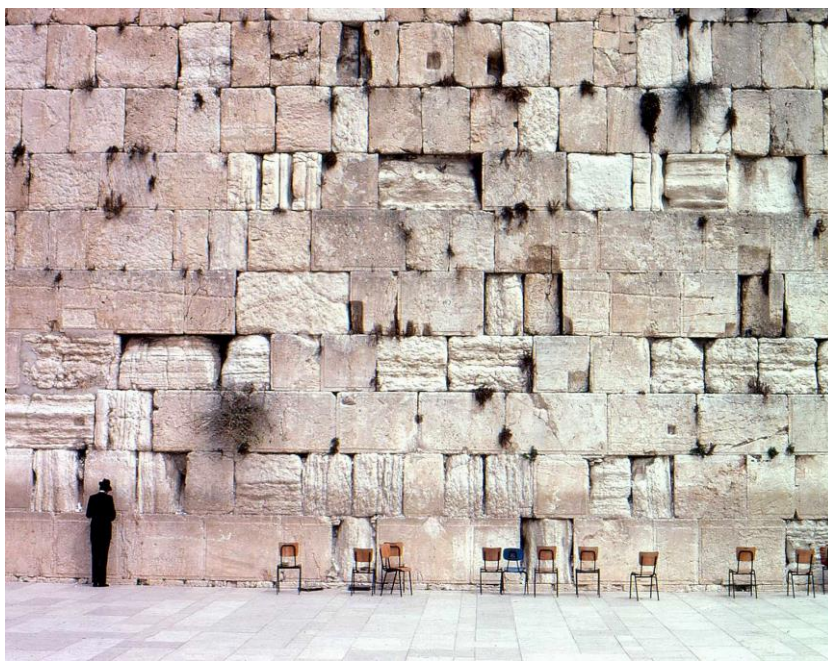
The Wailing Wall
